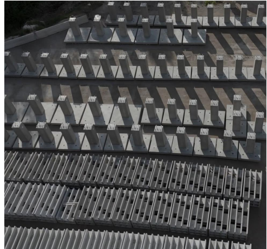
Troughs and foundations at the warehouse in Rättvik.
