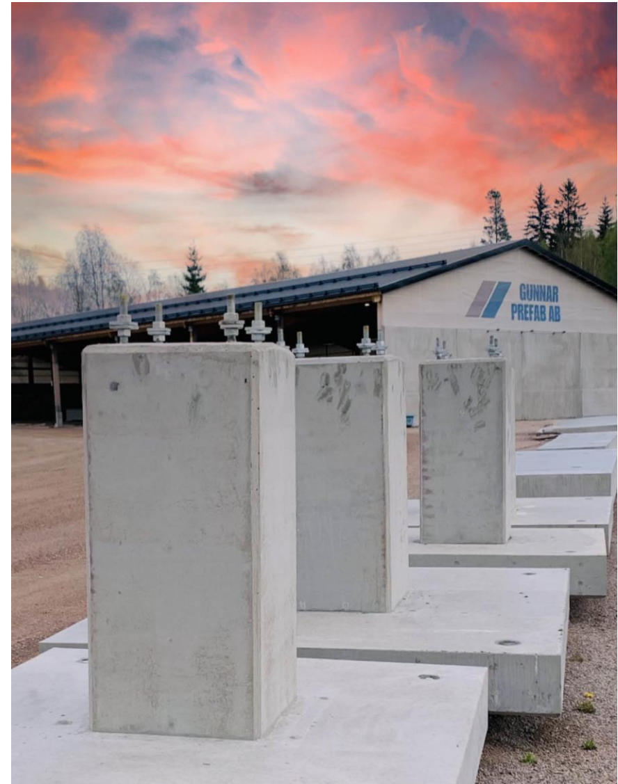
Switchyard foundations at the warehouse.
