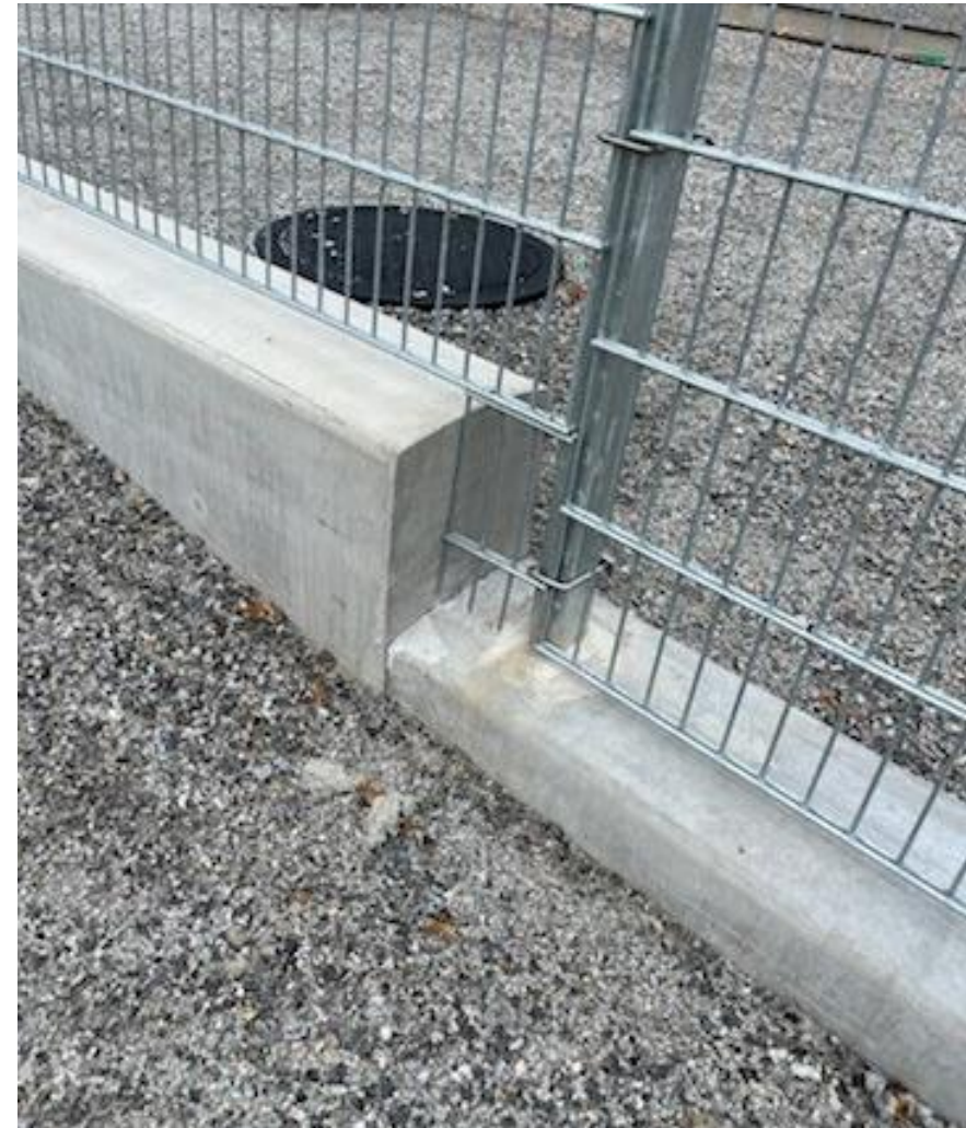
The anti-undermining barrier Protektor installed with a fence.
